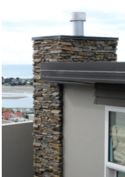
Corner stones returned to plaster cladding
